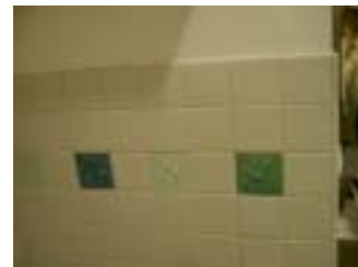
Toilet tiles made of crushed bottles
