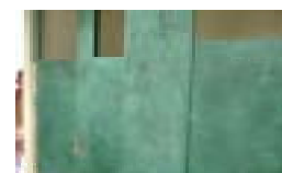
Toilet partitions made of crushed bottles
